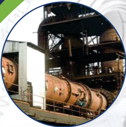
SPONGE IRON PLANT
