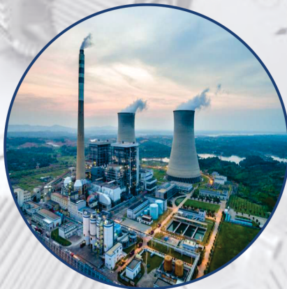
POWER THERMAL PLANT
